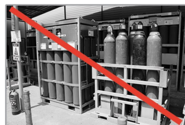
7/24 Own Nitrogen production (pic.1)
